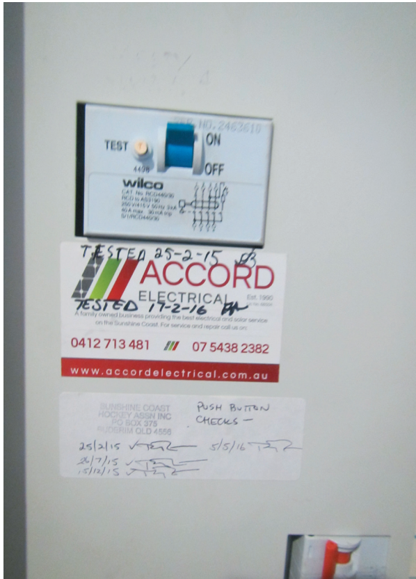
Secondary Breaker - Office: Will often trip as a secondary precaution when one of the other circuits breakers trip.
