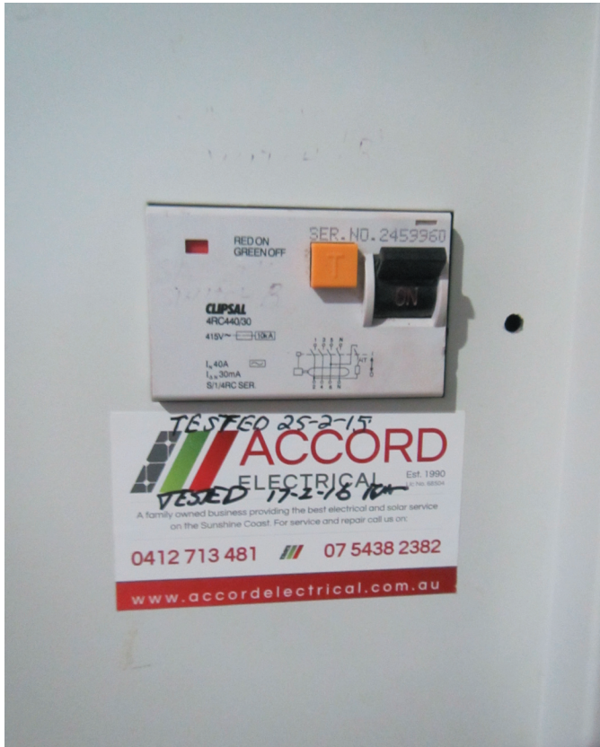
Switchboard Office: Main overload circuit breaker. Activation of this switch will see total loss of Power for the whole facility. If occurring while turf lights are on, turn lights off on computer panel and wait 20 minutes before re-turning lights on.
