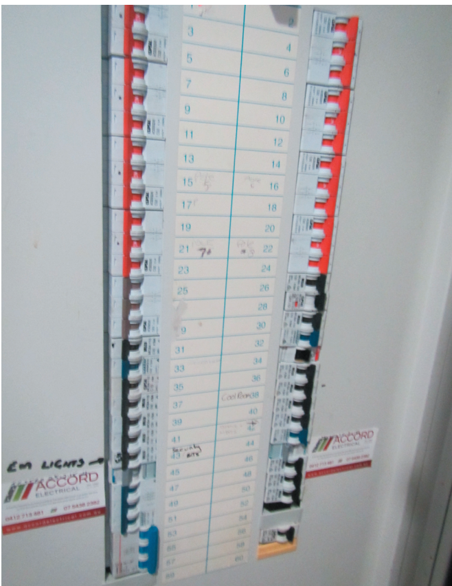
Circuits Breakers - Office: Breakers for all three circuits in clubhouse including turf lights. Running sheet for each individual switch and what it relates to is on the inside of the cabinet opposite the breakers.
